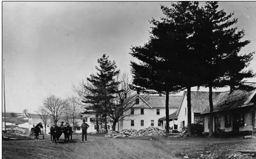
North Danville Village, with the old school in the background and Varney house (the large one on right). A flagpole is on the left, located where the new addition of Langmaid barn was built, circa 1900.
