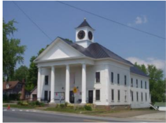
Danville Town Hall and Offices
