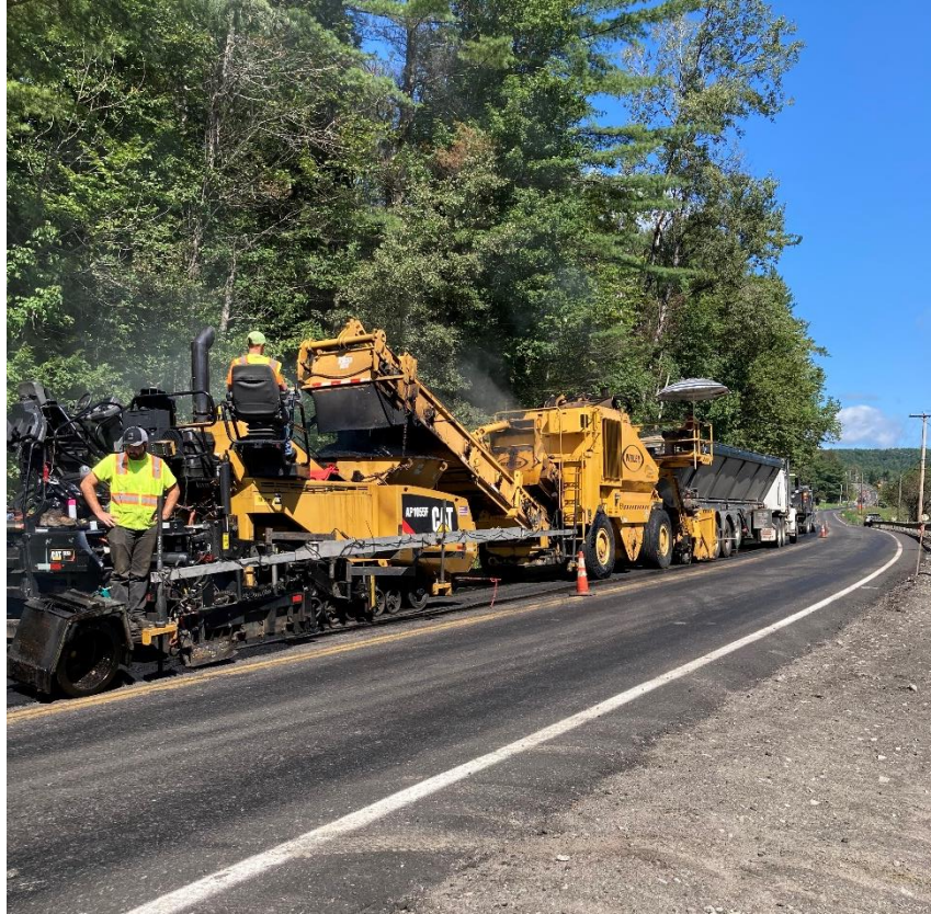
Crews paving the first layer of hot mix.
