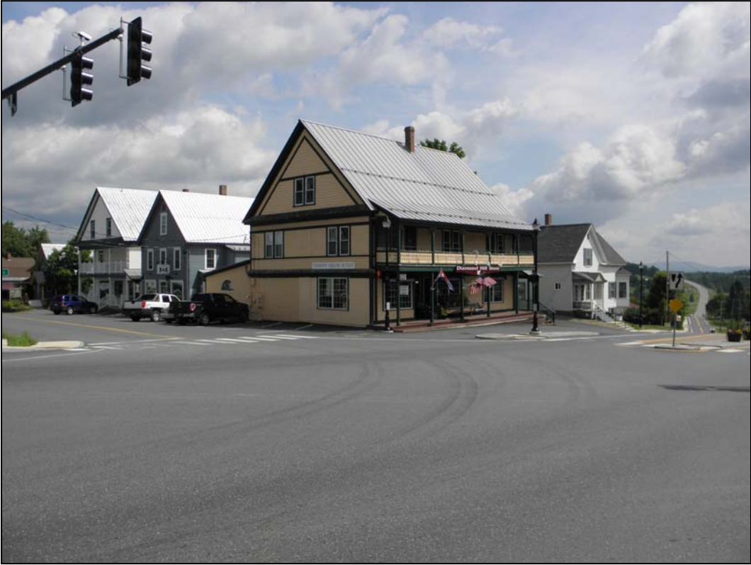
Photo 5. Structure 12, 11 US Route 2 (VHSS 0303-160, 8). View to the northeast.
