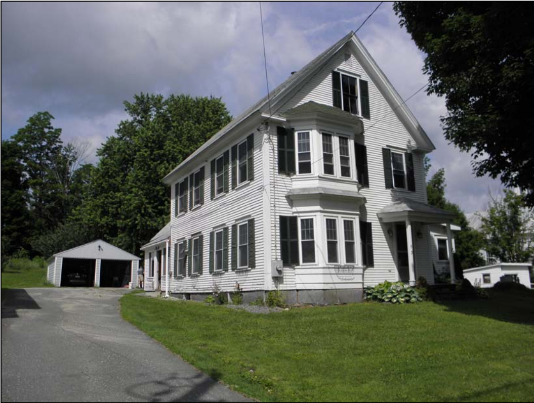
Photo 3. Structure 5, 53 Hill Street (VHSS 0303-160, 38). View to the west/northwest.
