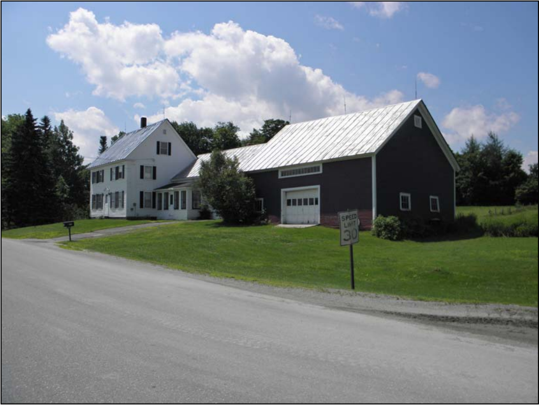
Photo 14. Structure 35, 478 Peacham Road (VHSS 0303-55). View to the southwest.
