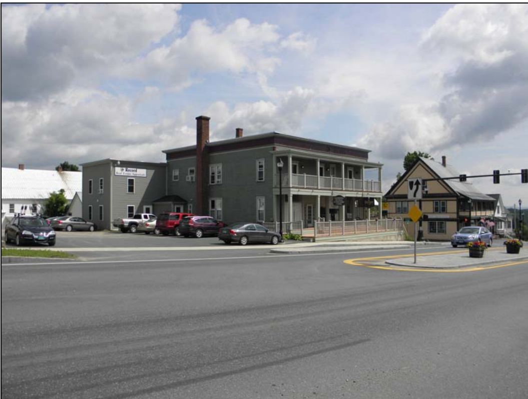
Photo 4. Structure 11, 10-12 US Route 2 (VHSS 0303-160, 33). View to the northeast.
