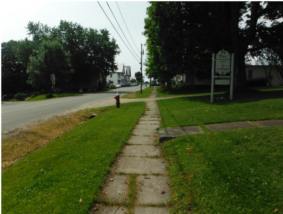
Existing Sidewalk along Hill Street
