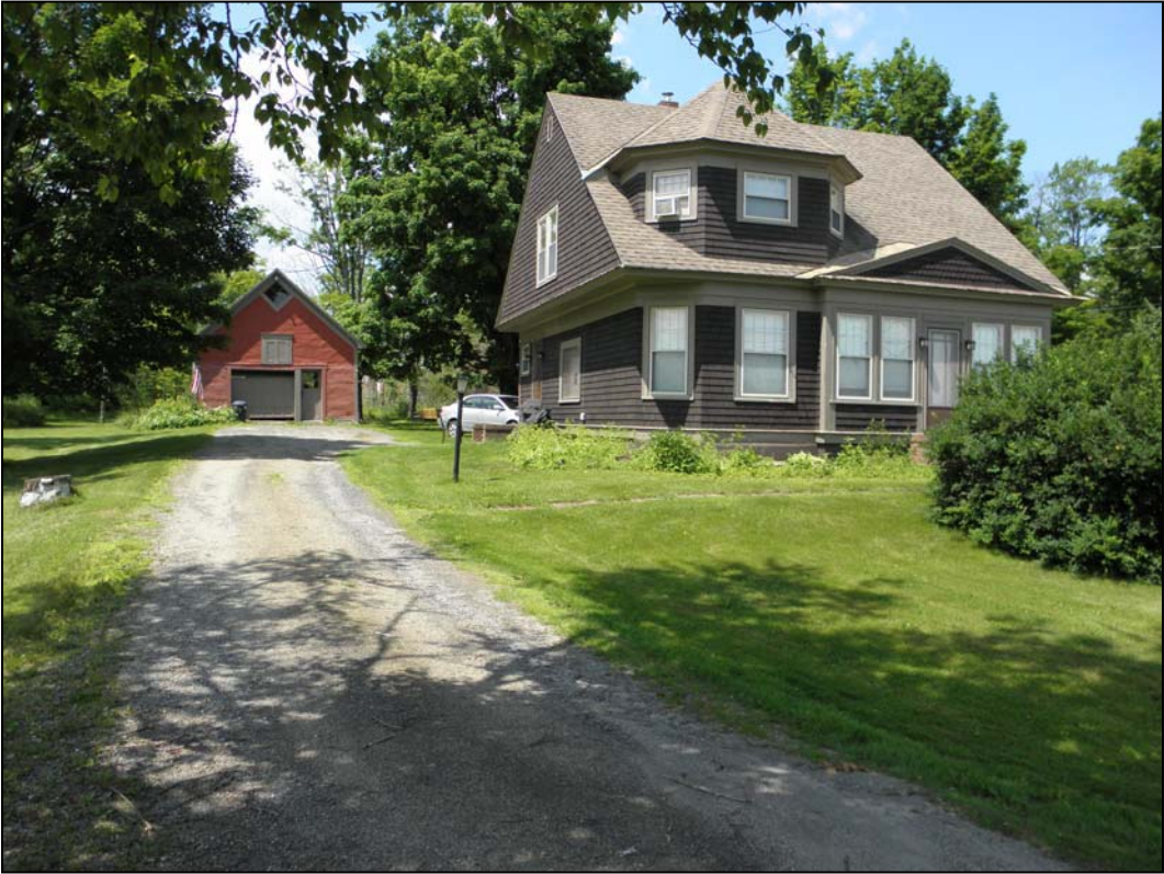
Photo 13. Structure 32, 428 Peacham Road (VHSS 0303-60). View to the west.
