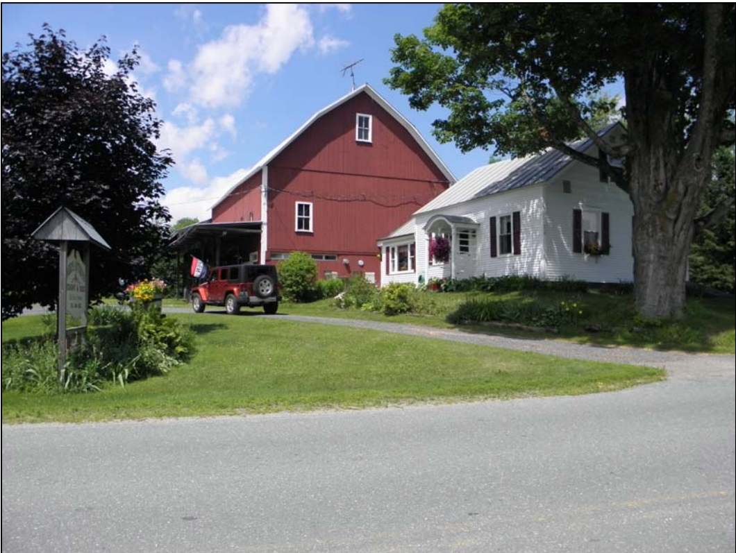
Photo 12. Structure 30, 378 Peacham Road (VHSS 0303-69). View to the northwest.
