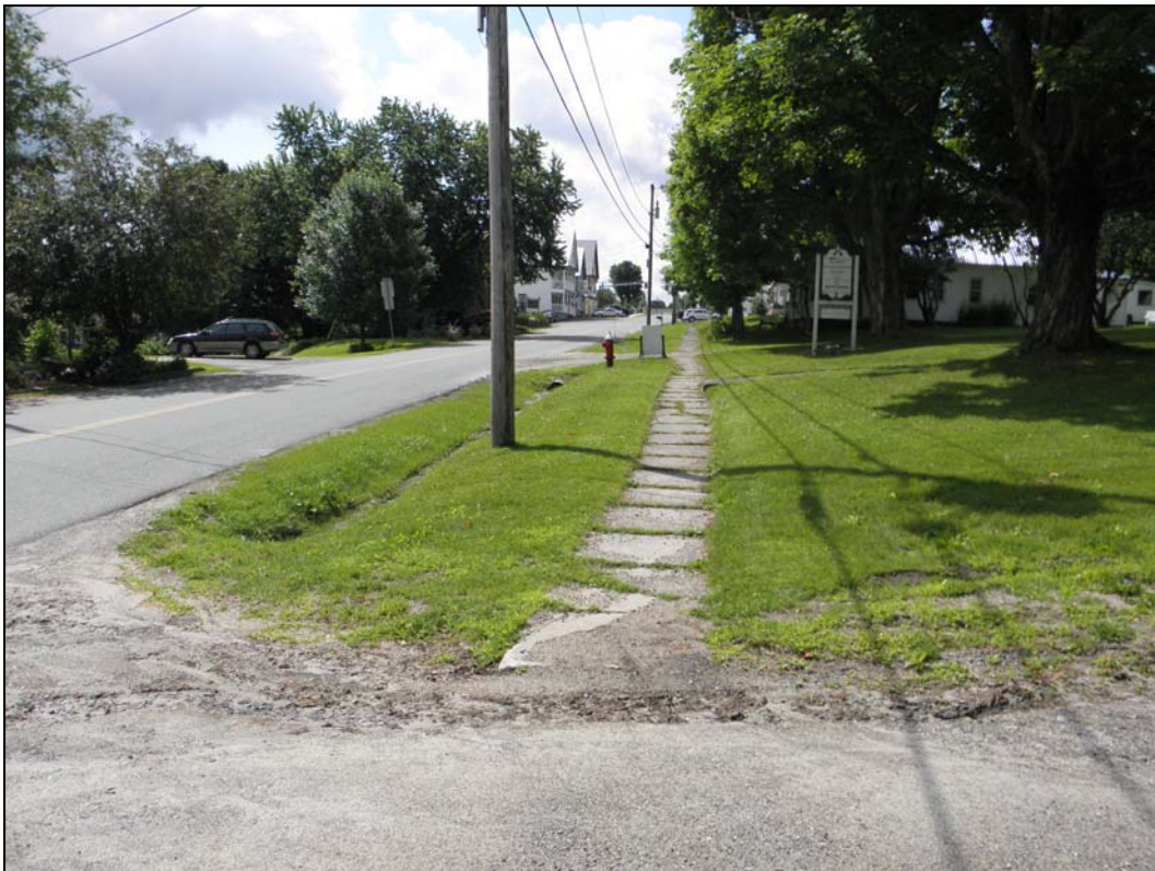
Photo 19. Existing sidewalk along the west side of Hill Street. View to the south.
