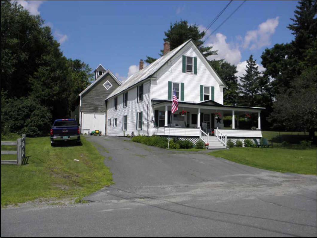
Photo 10. Structure 21, 218 Peacham Road (VHSS 0303-163, 12). View to the northwest.
