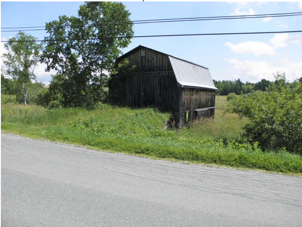
Photo 16. Structure 31, unidentified address on Peacham Road. A gambrel-roofed barn not associated with a standing house. View to the northeast.
