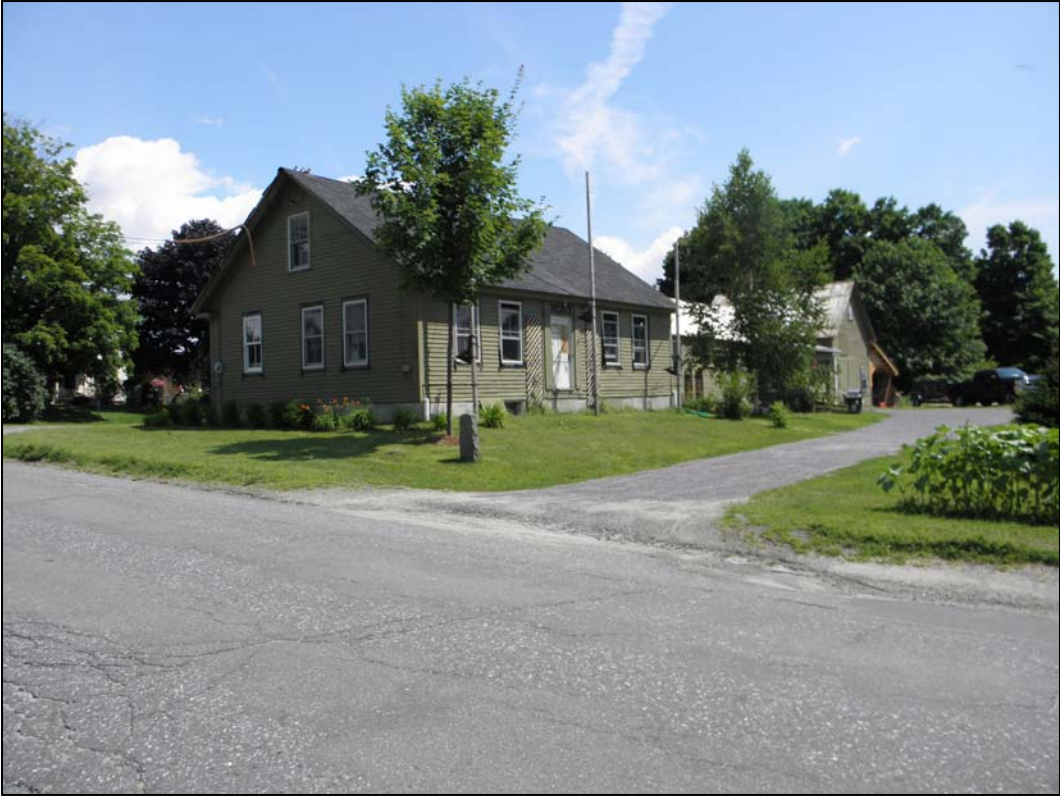
Photo 7. Structure 13, 123 (?) Peacham Road (VHSS 0303-163, 2). View to the northeast.
