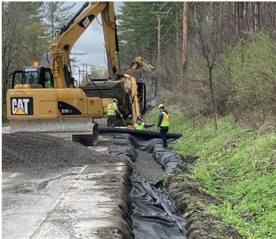
Crews working on underdrain.
