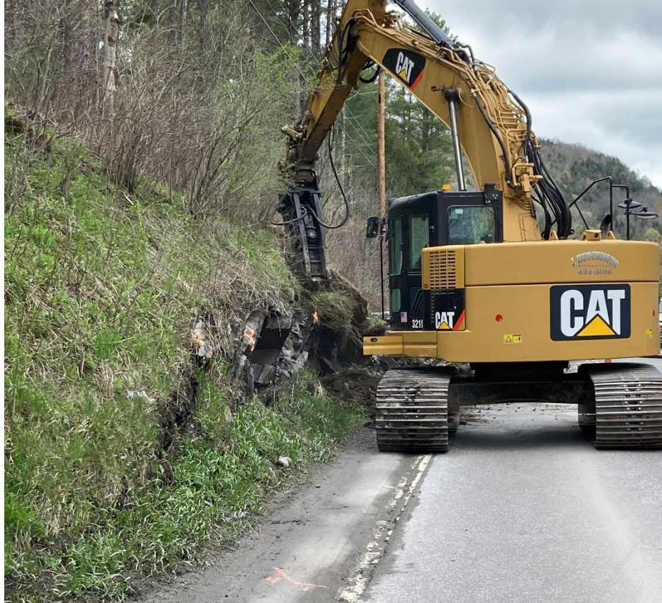
Ledge removal on a slope.
