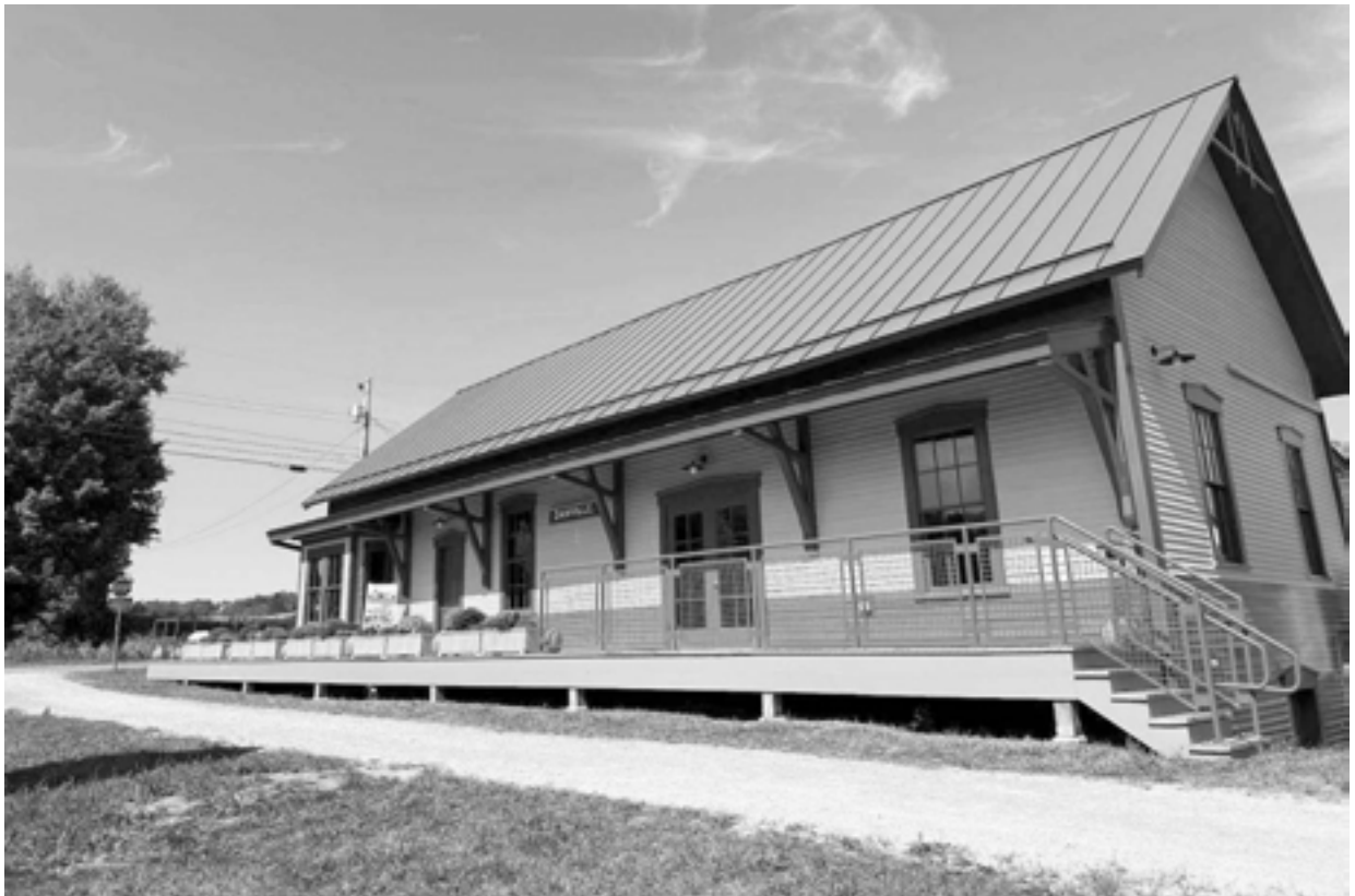
Danville's newly renovated Train Station. Photo credit Chelsea Hewitt.
