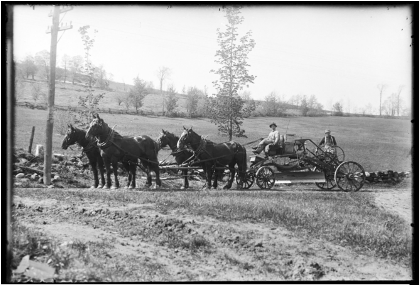
A four-horse hitch road grader. The driver looks a little cavalier with his legs crossed. (Harold Hatch collection)
