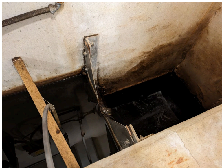
Figure 2-14: Effluent V-Notch Weir
