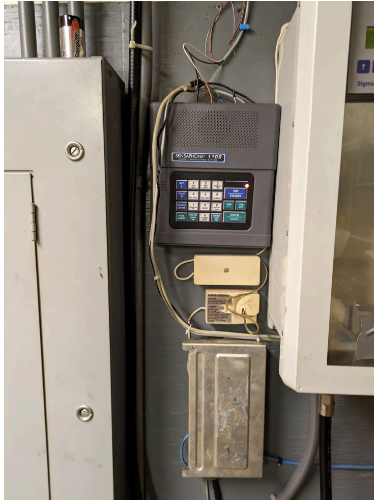
Figure 2-13: Alarm Autodialer
