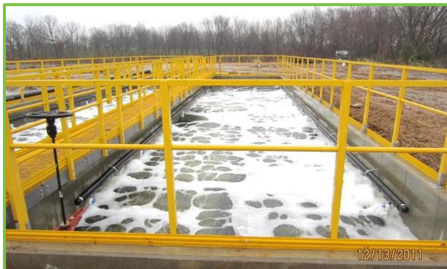
Lemna Polishing Reactor (LPR)
