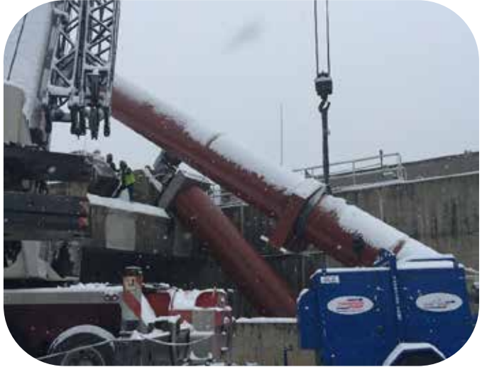
Screw Pump Installation in St. Johnsbury
