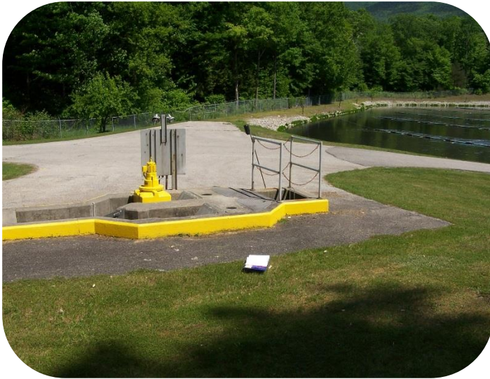
Flow Control Structure
