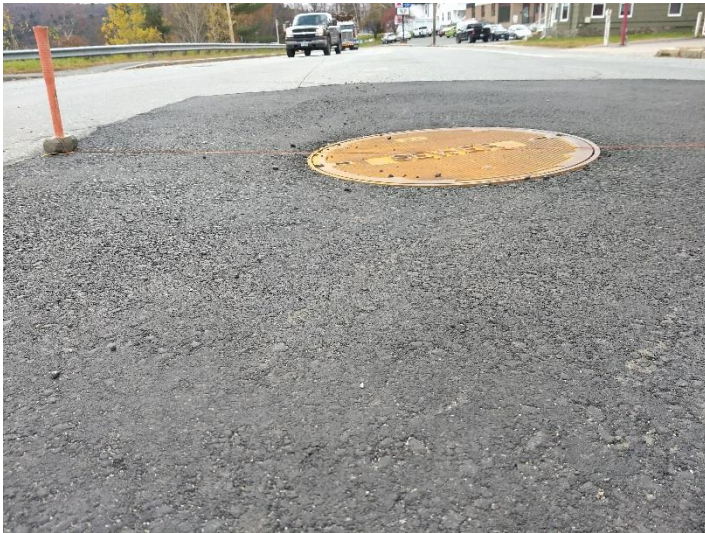
A new manhole on Union Street
