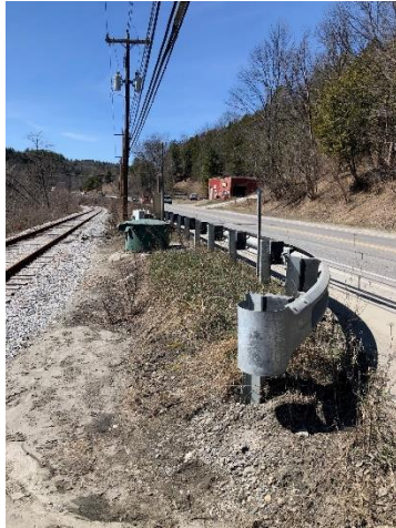
Existing Pneumatic Ejector Station
