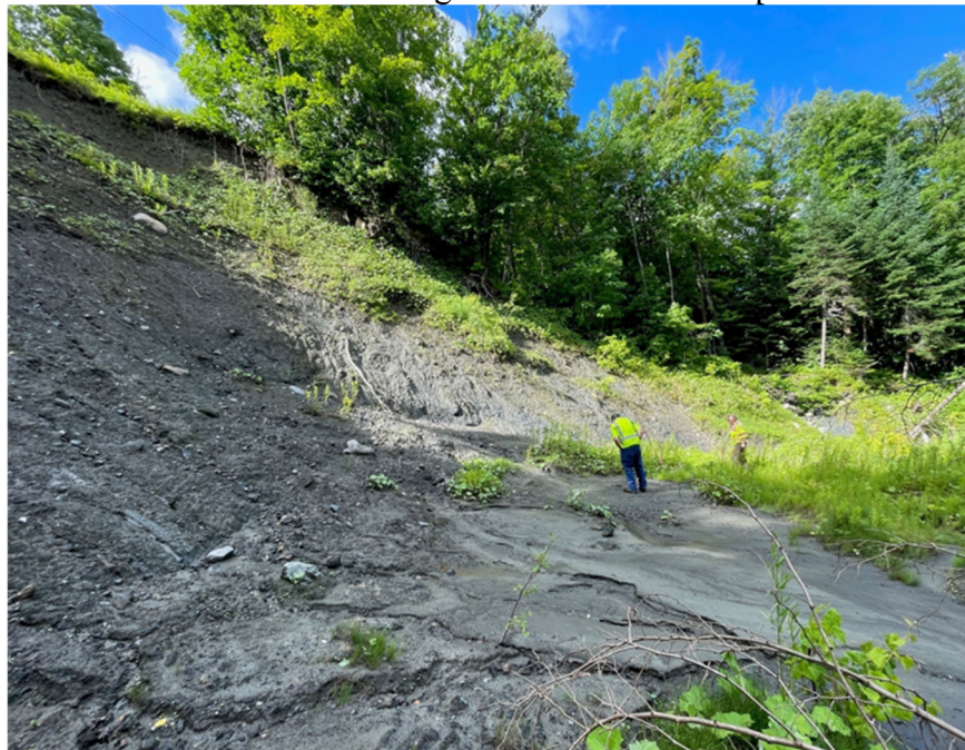
Photo 1: Looking west at the toe of slope
